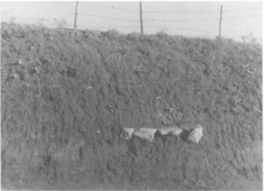
Figure 5.5 Limestone paving of a road leading from the Via Flaminia to the Tiber Source: British School at Rome Archive, John Ward Perkins Collection
