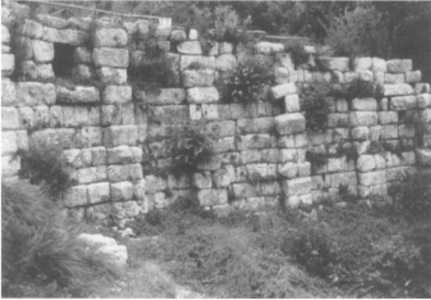
Figure 14.5 A road viaduct maintains a flat surface for the traveller across a valley; Ponte del Diavolo on the Via Salaria
