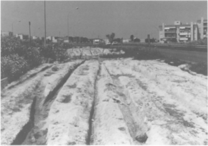
Figure 5.2 Eroded road surface of the Via Traiana at Monopoli
