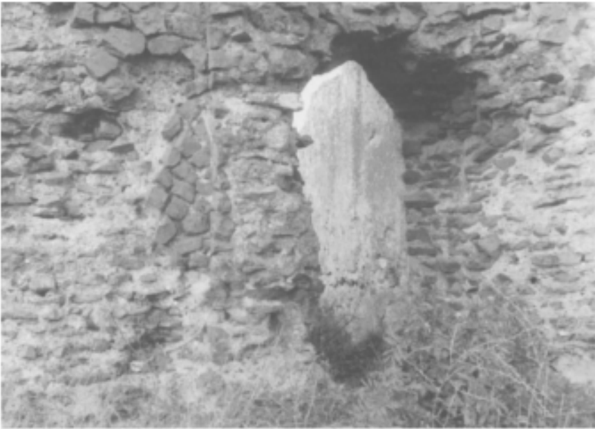
Figure 5.7 Selce Opus Reticulatum : south Etruria
